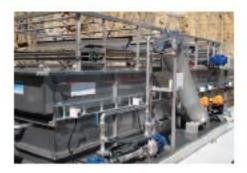
For economies of size, sludge concentration and efficiency of separation of wide ranging solids densities, DAF is the often the most appropriate process to employ for many trade waste applications.
